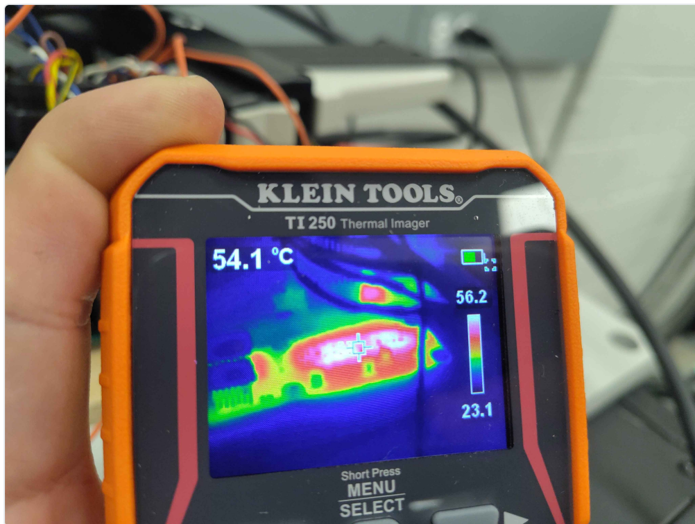
Gate-driver area, the hottest point during the run
